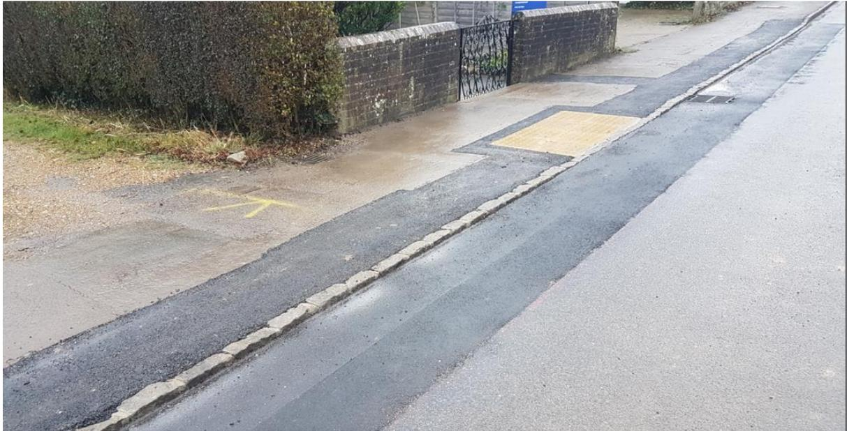
Inspection shows that whilst the level of the protective kerb has been raised as expected along most of the excavated edge, at the section of dropped kerb tactile paving, the road tarmac surface now almost matches the level of the tactile paving and the expected 25mm lip has not been achieved.
